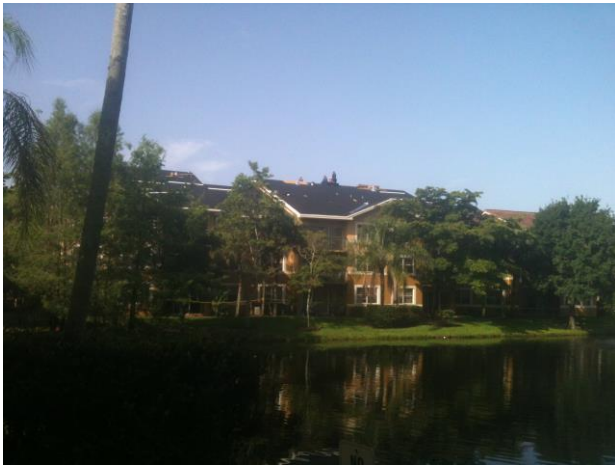
DURING TEAR OFF - 2013
