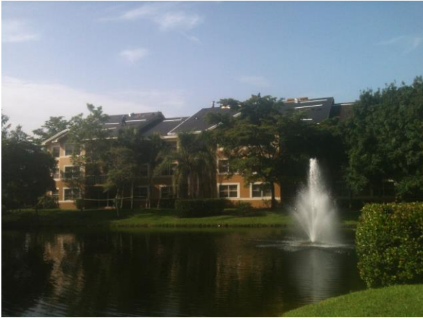
TEAR OFF OLD ROOF - 2013
