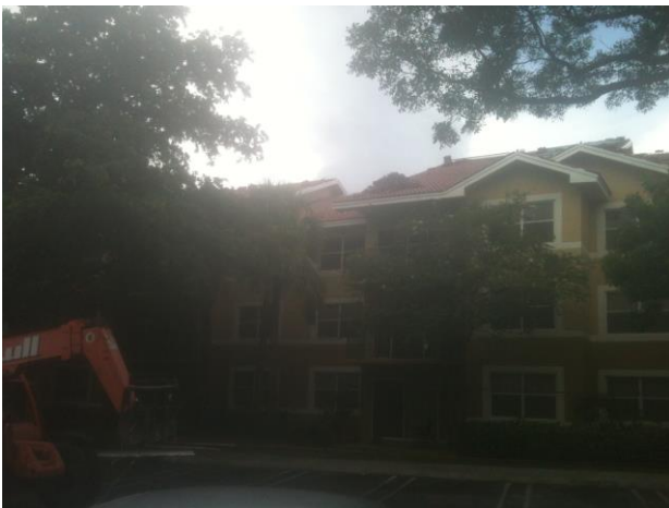
TILE LOAD AND INSTALL - 2013
