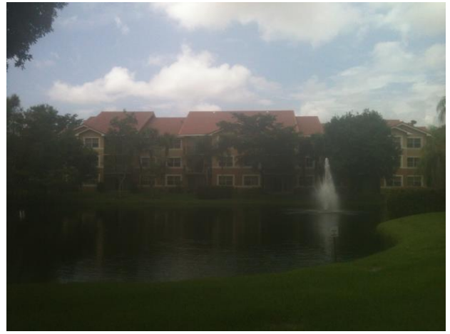
NEW ROOF COMPLETE - 2013
