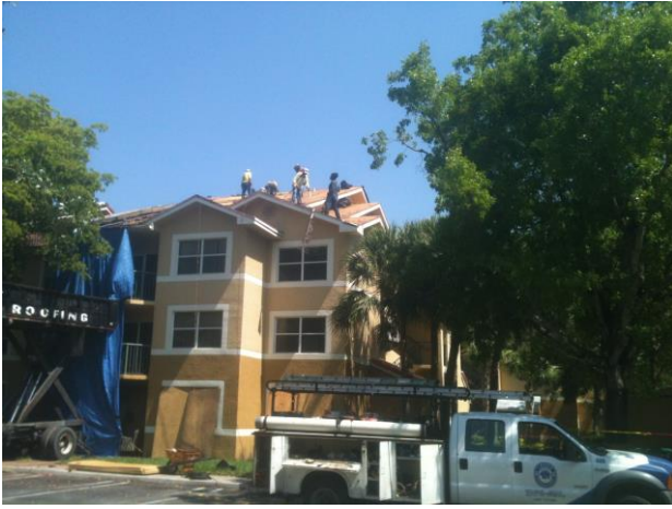
TEAR OFF OLD ROOF - 2013
