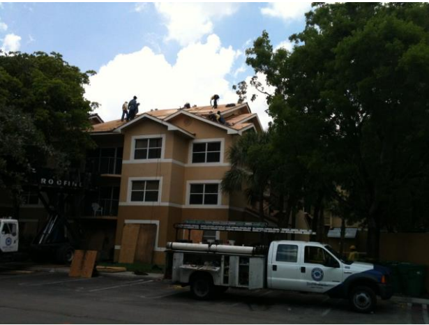
DURING TEAR OFF - 2013
