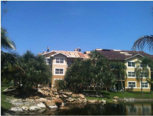
DURING TEAR OFF - 2013
