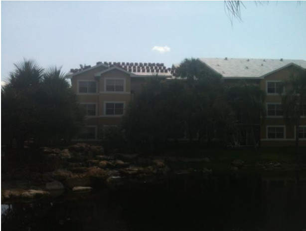
TILE LOADED FOR INSTALL - 2013
