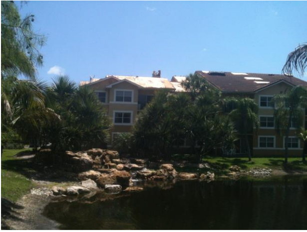
TEAR OFF OLD ROOF - 2013
