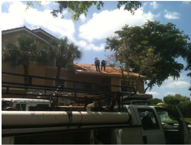
DURING TEAR OFF - 2013
