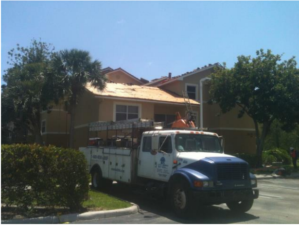
TEAR OFF OLD ROOF - 2013
