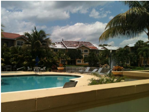
TILE LOADED FOR INSTALL - 2013
