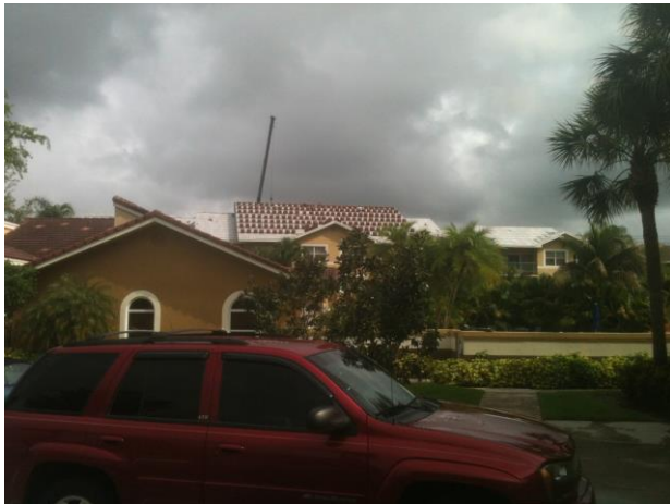
TILE LOADED FOR INSTALL - 2013
