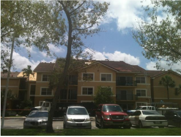
TEAR OFF OLD ROOF - 2013
