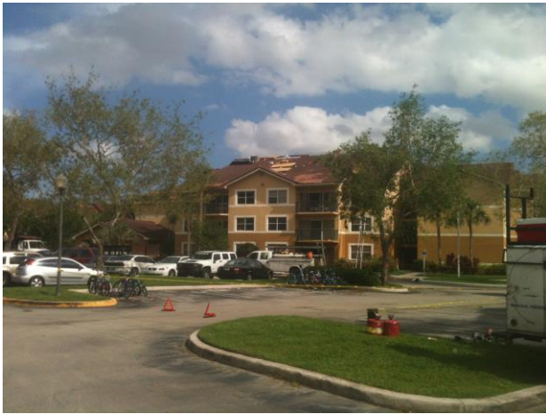
DURING TEAR OFF - 2013
