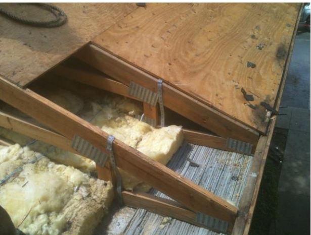
TRUSS STRAP CONFIGURATION - 2013
