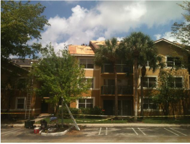
TEAR OFF OLD ROOF - 2013
