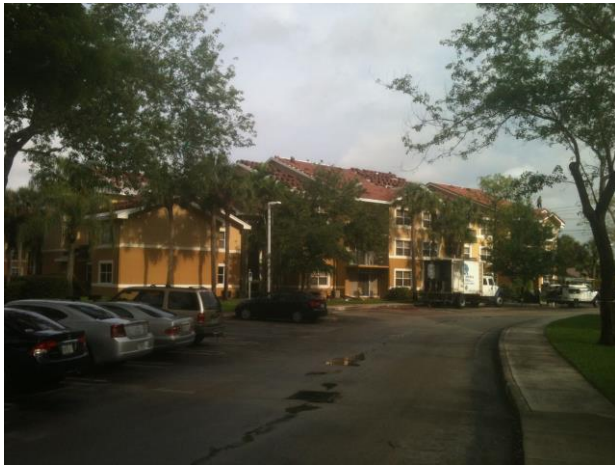
TILE LOADED FOR INSTALL - 2013
