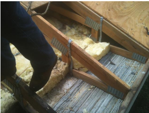
TRUSS STRAP CONFIGURATION - 2013
