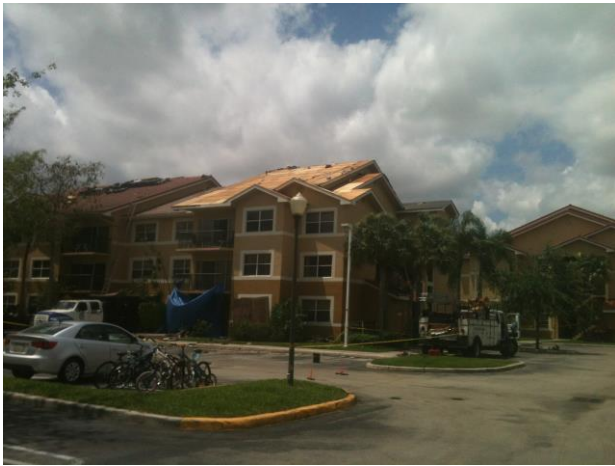
DURING TEAR OFF - 2013
