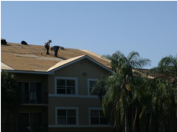
DURING TEAR OFF - 2013
