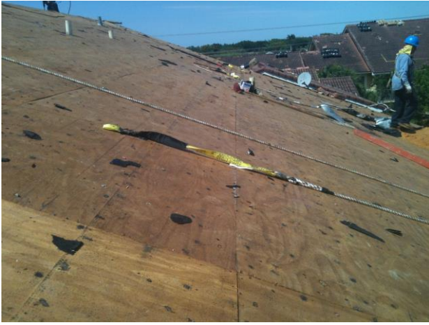
TEAR OFF OLD ROOF - 2013
