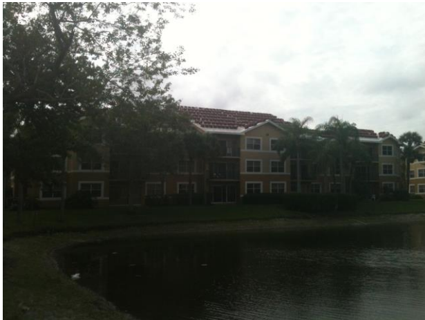
TILE LOADED FOR INSTALL - 2013
