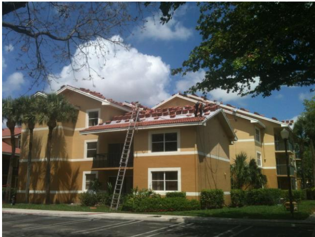
TILE LOADED FOR INSTALL - 2013
