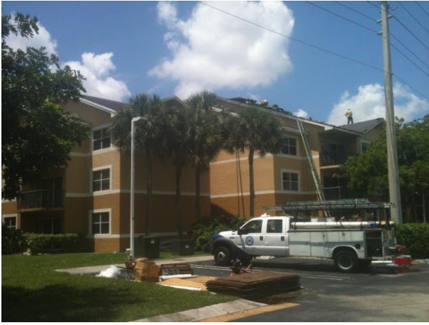
TEAR OFF OLD ROOF - 2013
