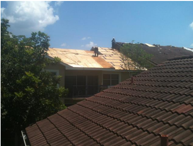
TEAR OFF AND SWR INSTALL - 2013
