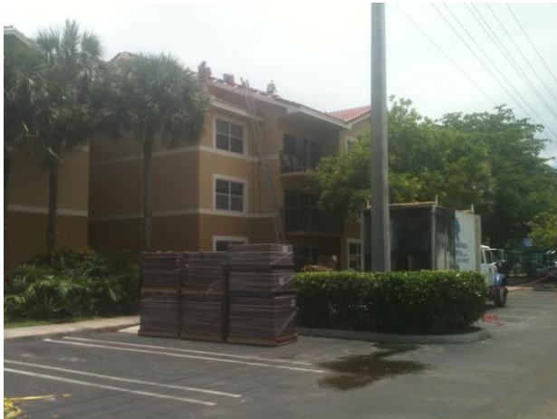
TILE LOADED FOR INSTALL - 2013
