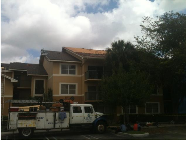
TEAR OFF OLD ROOF - 2013
