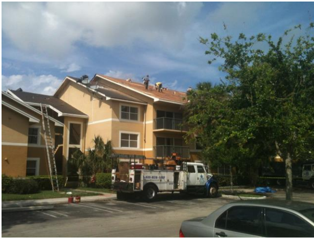
DURING TEAR OFF - 2013
