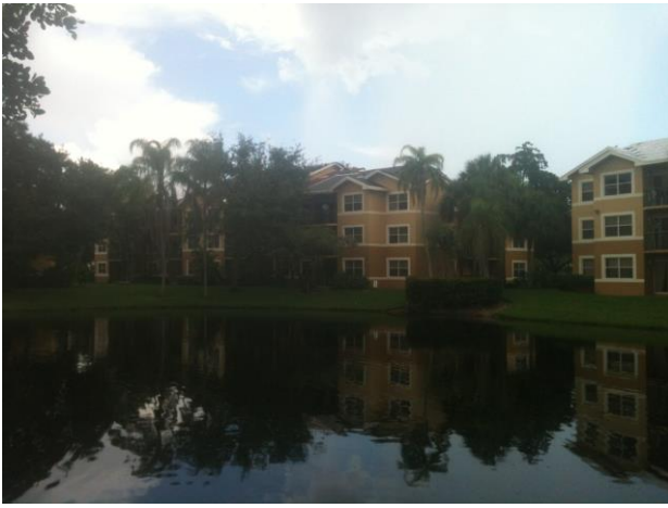
TEAR OFF OLD ROOF - 2013
