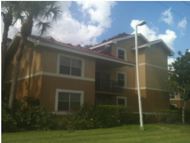
TILE LOADED FOR INSTALL - 2013
