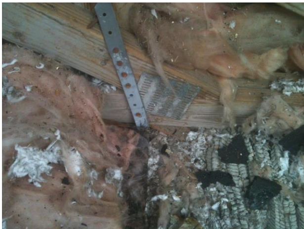
TRUSS STRAP CONFIGURATION - 2013
