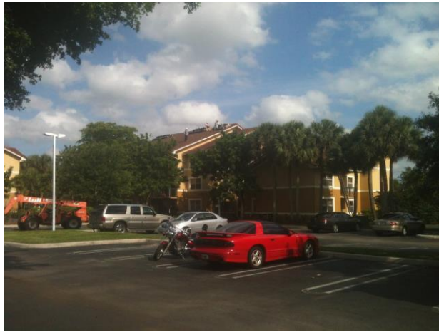
DURING TEAR OFF - 2013
