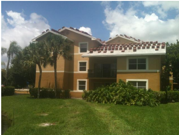
TILE LOADED FOR INSTALL - 2013
