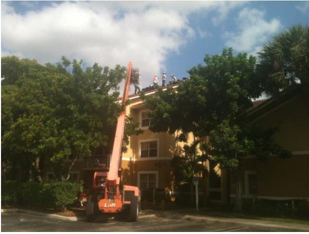
TEAR OFF OLD ROOF - 2013
