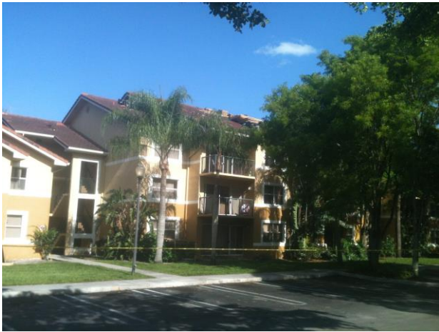
DURING TEAR OFF - 2013
