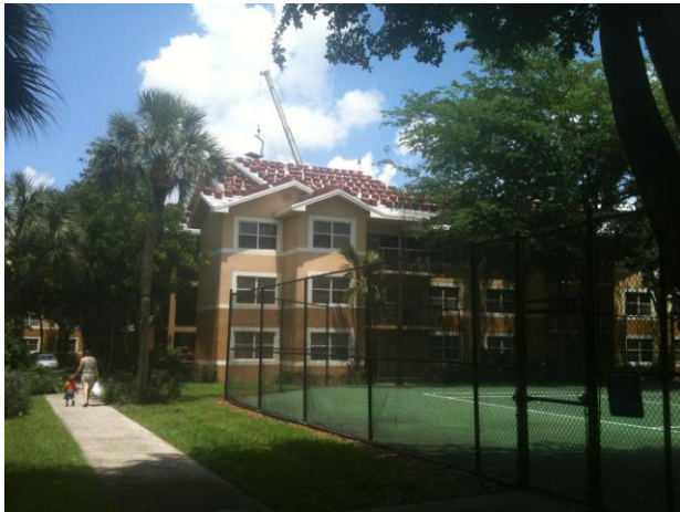
TILE LOADED FOR INSTALL - 2013
