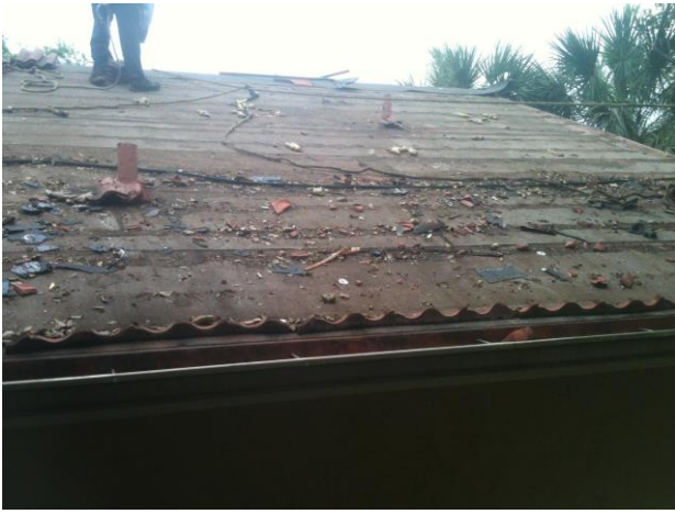
TEAR OFF OLD ROOF - 2013
