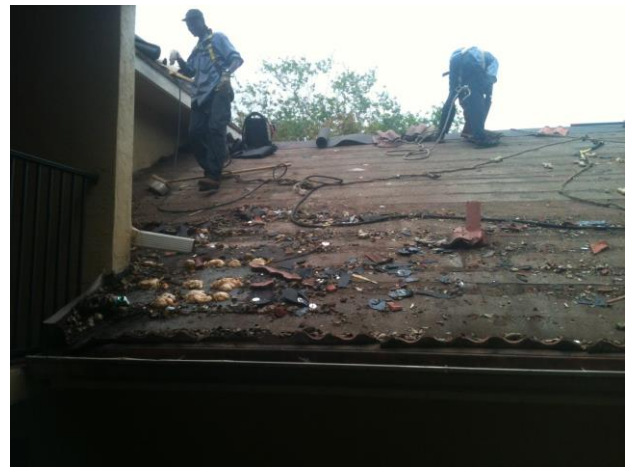
DURING TEAR OFF - 2013
